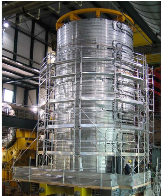
Figure 14 – The cold mass mounted vertically before integration and insertion in the vacuum chamber.
